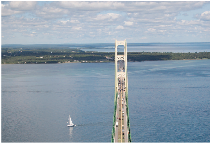
On Labor Day, thousands will enjoy the thrill of a lifetime by strolling the Mighty Mac. During peak summertime season, the bridge transports more vehicles across the Straits of Mackinac in a single month than the ferry system did in an entire year when it was in operation. PHOTO BY JIM AKANS
